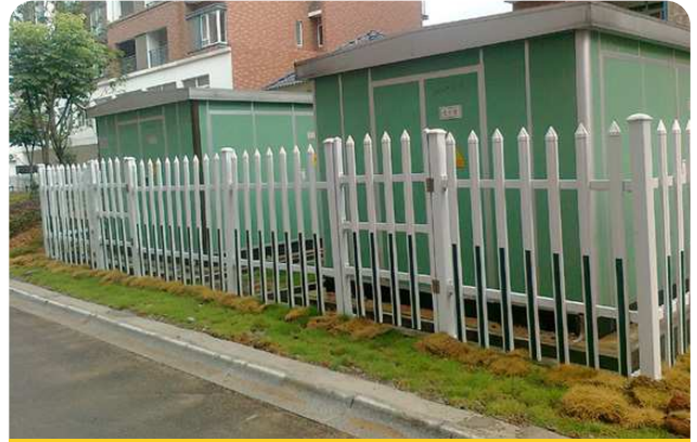
Power Station Fencing
