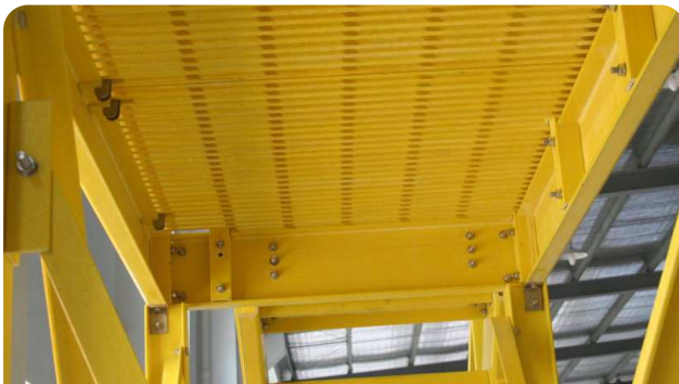
FRP Channel Ladders Supports
