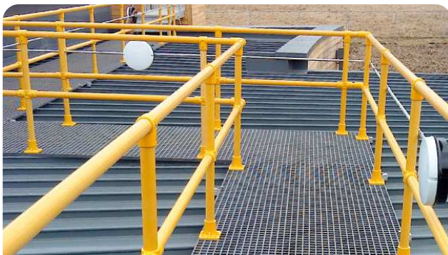
Roof walkway Guardrail
